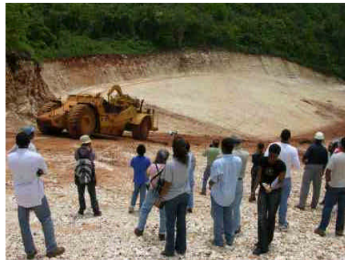
Mined out pit being topsoiled
