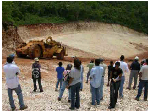
Mined out pit being topsoiled
